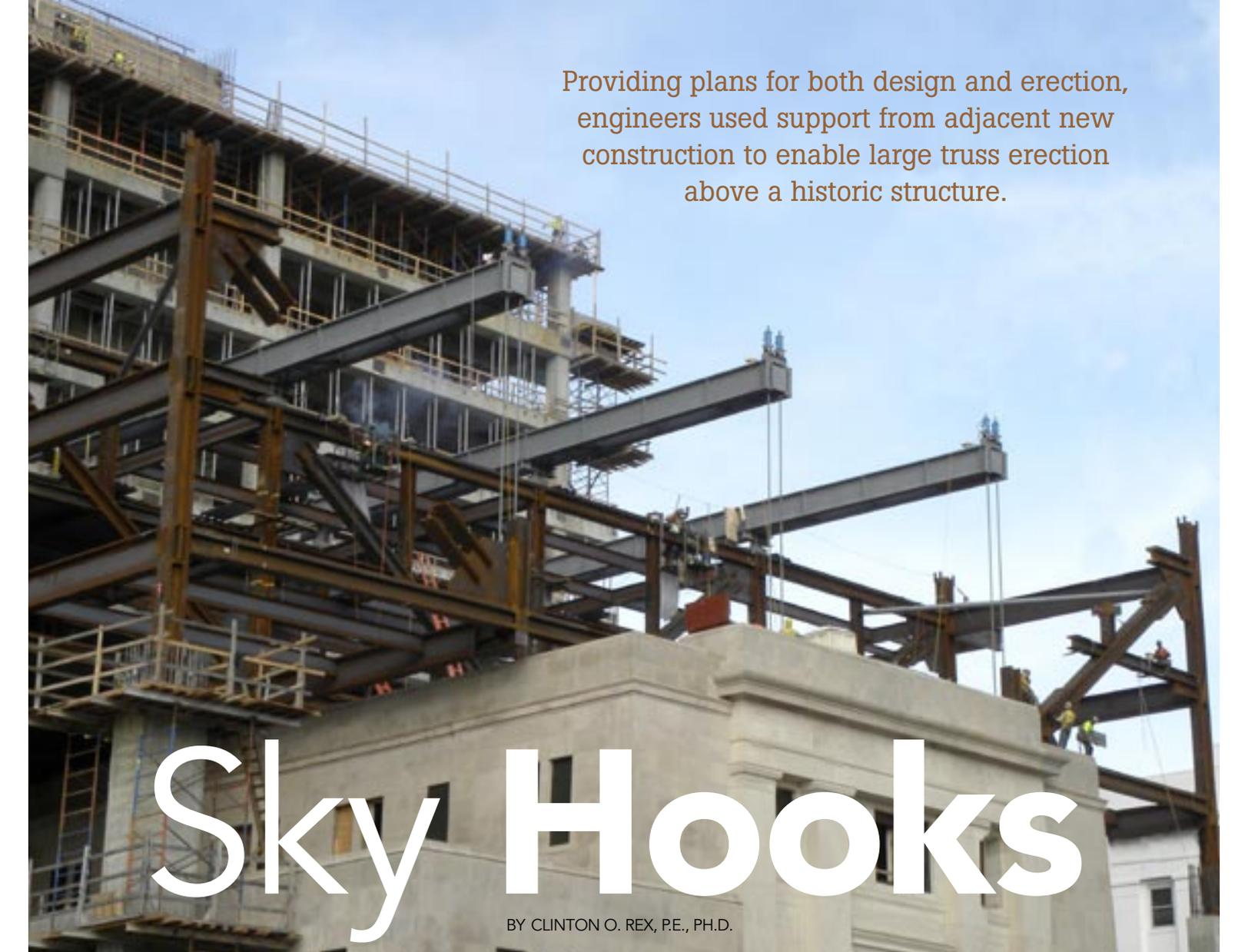
Providing plans for both design and erection, engineers used support from adjacent new construction to enable large truss erection above a historic structure.
